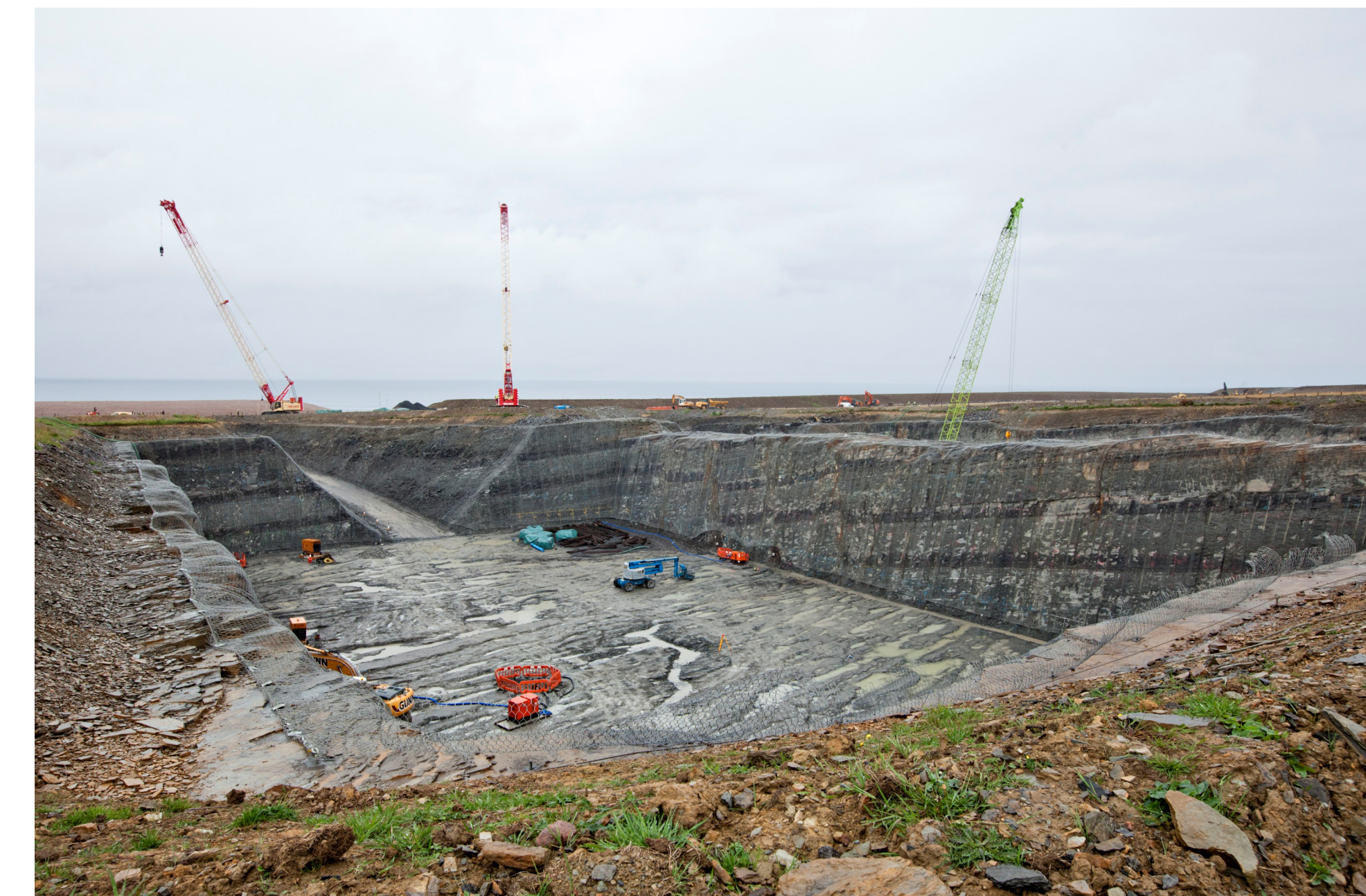
Vault excavation during construction
